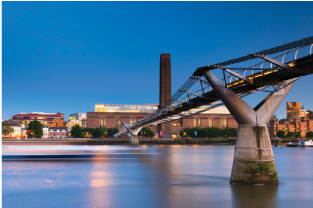
Figure 18.29: The 'wobbly' Millennium Bridge in London was closed for nearly two years to correct problems caused by resonance.
